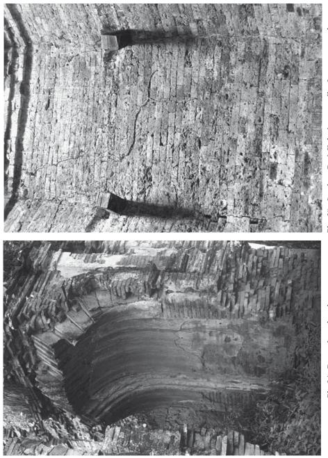
Ph. 35. Sambor Prei Kuk, inner wall of an octagonal tower made of brick, with sandstone hooks supporting the ceiling beams.
