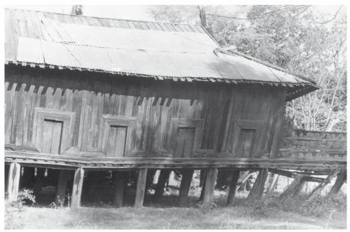
Ph. 25. Mandalay, Burma, longitudinal façade of a building on partially buried piles.
